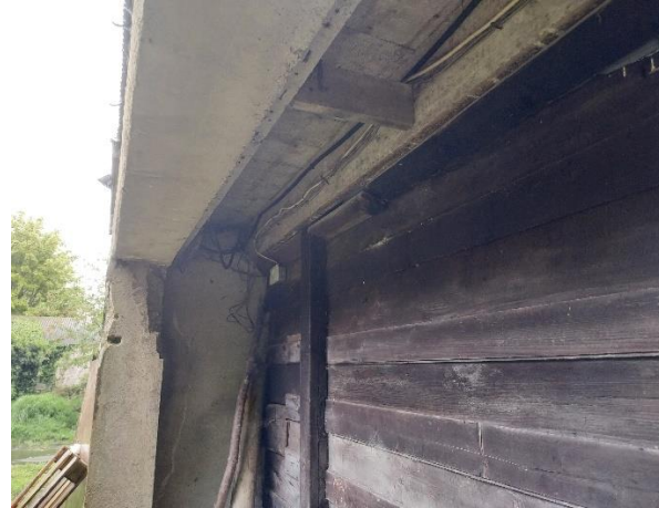
Plate 4 - Eastern side – Holes in wood and gaps around entrance
