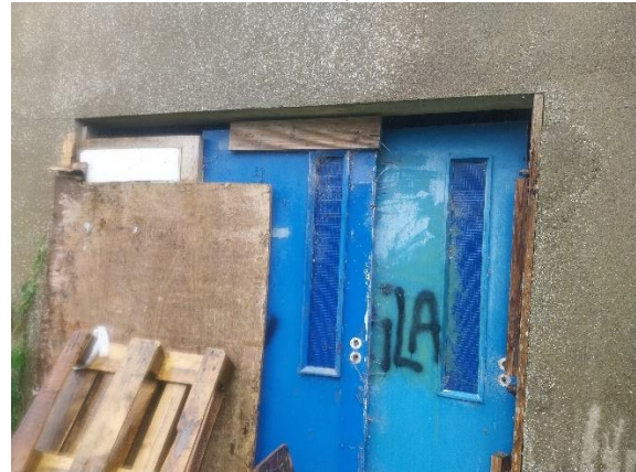
Plate 6 – Eastern side – Gaps around entrance
