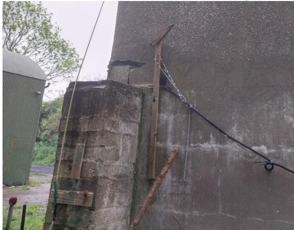
Plate 3 – Northern side – Holes in cladding
