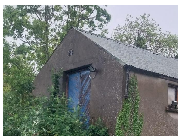
Plate 8 – Southern side – Gaps under roof
