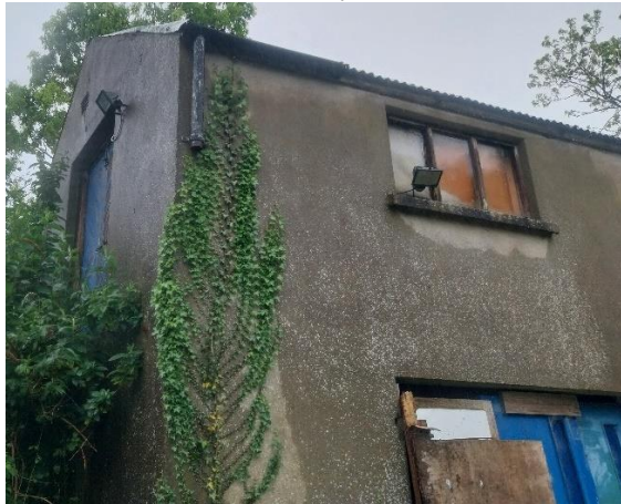
Plate 9 – Eastern side – Gaps under roof
