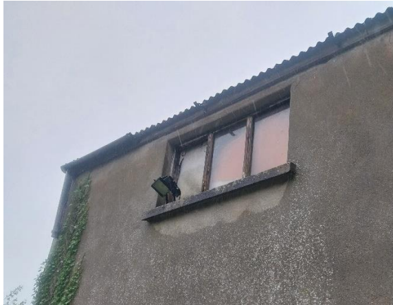
Plate 7 Eastern side – Crevices around window
