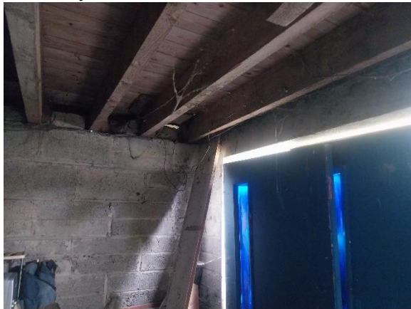
Plate 15 – Ground floor, southern room – Gaps between joists
