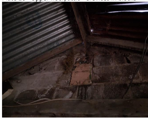
Plate 20 - Upper floor/attic - Crevices in blocks
